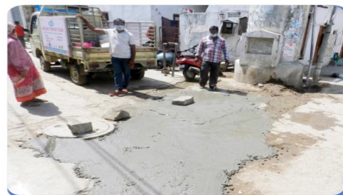
Repair Road at Masjid Circle Vemukunta (After)
