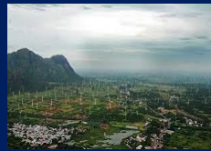
Muppandal Wind Farm: 1,500MW
