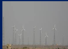
Jaisalmer Wind Park: 1,064MW
