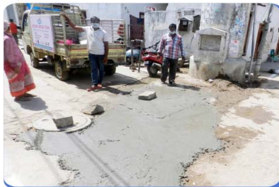
Repair Road at Masjid Circle Vemukunta (After)
